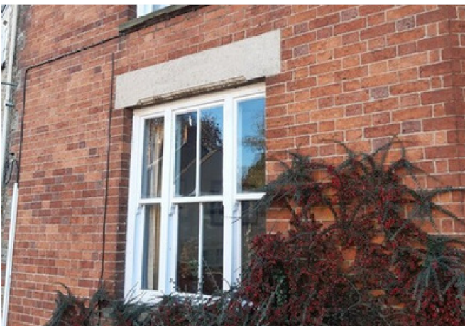
Church Rise, Flemish bond brickwork at the entrance to Church Lane.
