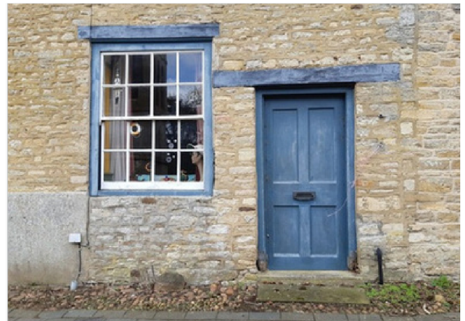
Window and door at 3 High Street.
